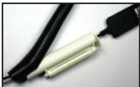
▲ CABLE ARMOR Threading the armor with cable.
